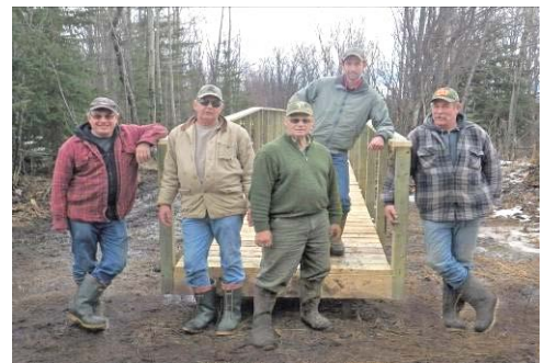
Construction crew L to R Barry Sideroff, Peter Martin, Don Nelson, Colter Grinde, & Bruce Popesc
